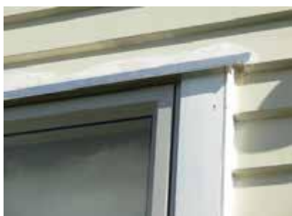
Aluminium window retrofitted into existing wall with new head flashing, boxed trim and scriber.
