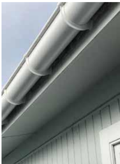
Gutter in good condition
