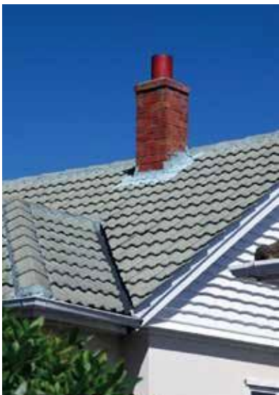
Heavyweight roof (concrete tiles).
