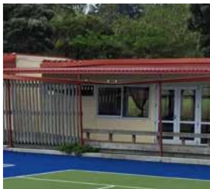
Gutter requiring urgent repair
