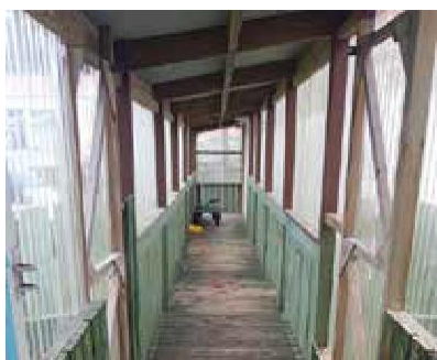
Translucent sheeting in corridor – a high impact area
