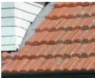
Lead flashing to clay tiles
