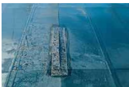
Patch repair to joint
