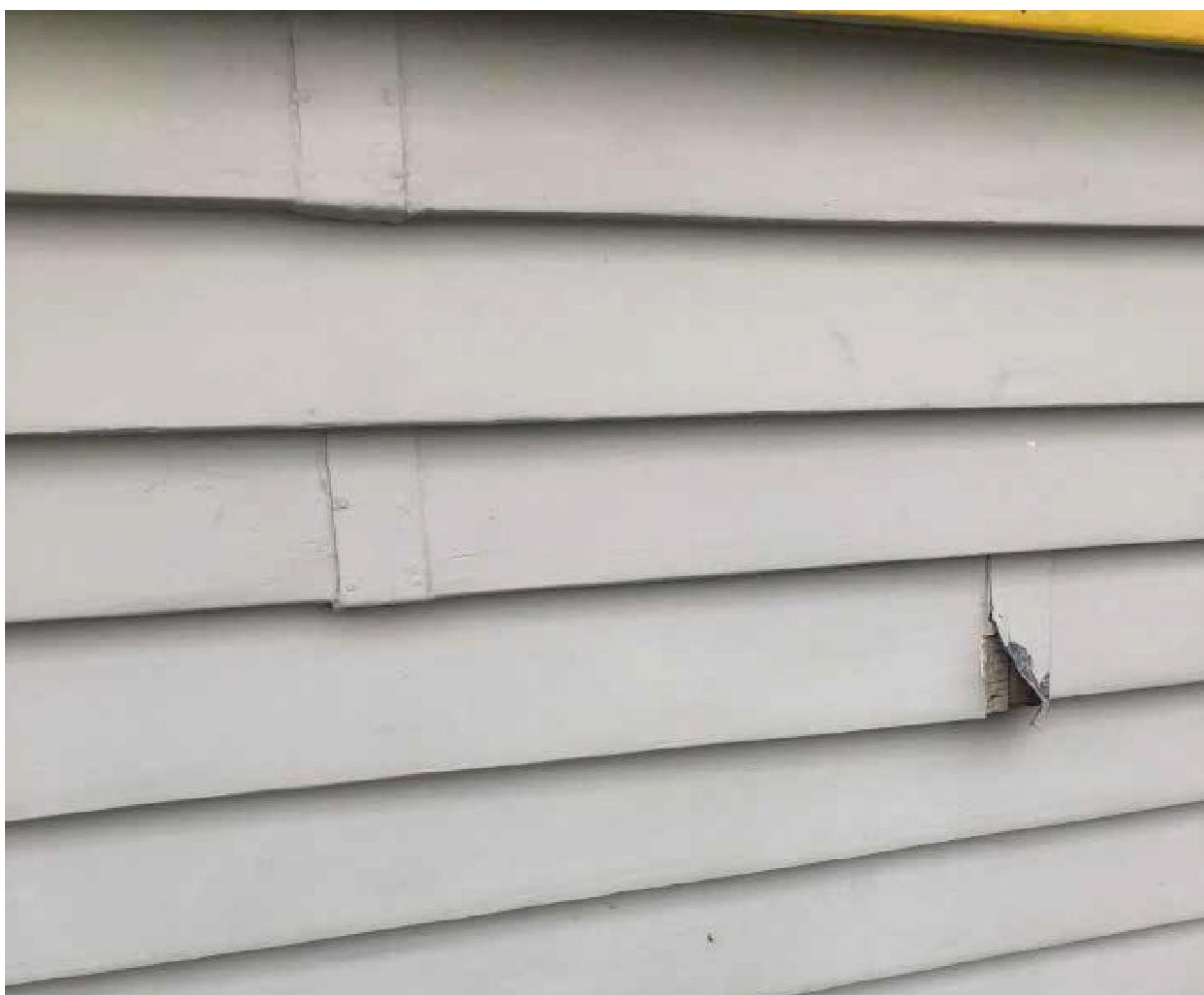
Repair soaker flashing at weatherboard junction
