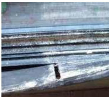
Chalking on aluminium joinery
