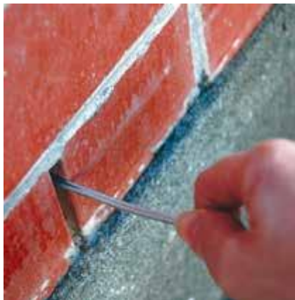
Cleaning drainage slots at bottom of veneer to allow for drainage of cavity
