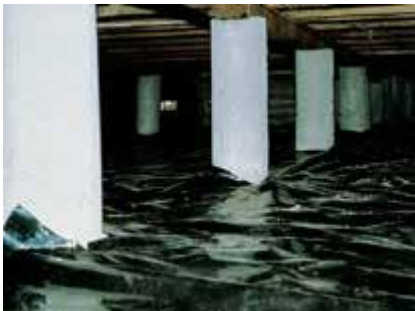
Subfloor polythene (taped at joints) to reduce rising damp
