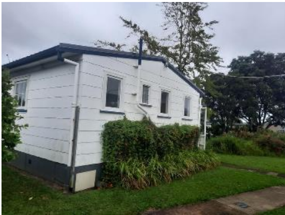
Plants affecting the performance of the cladding
