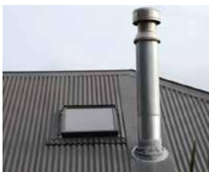
Flue stays not installed
