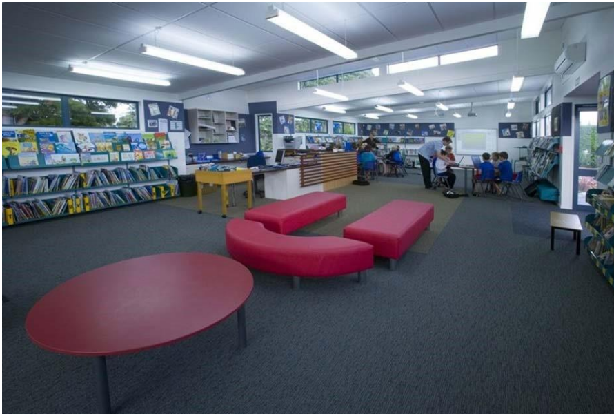
Figure 28: Library: a mix of side lighting, clerestory lighting and suspended luminaires.
