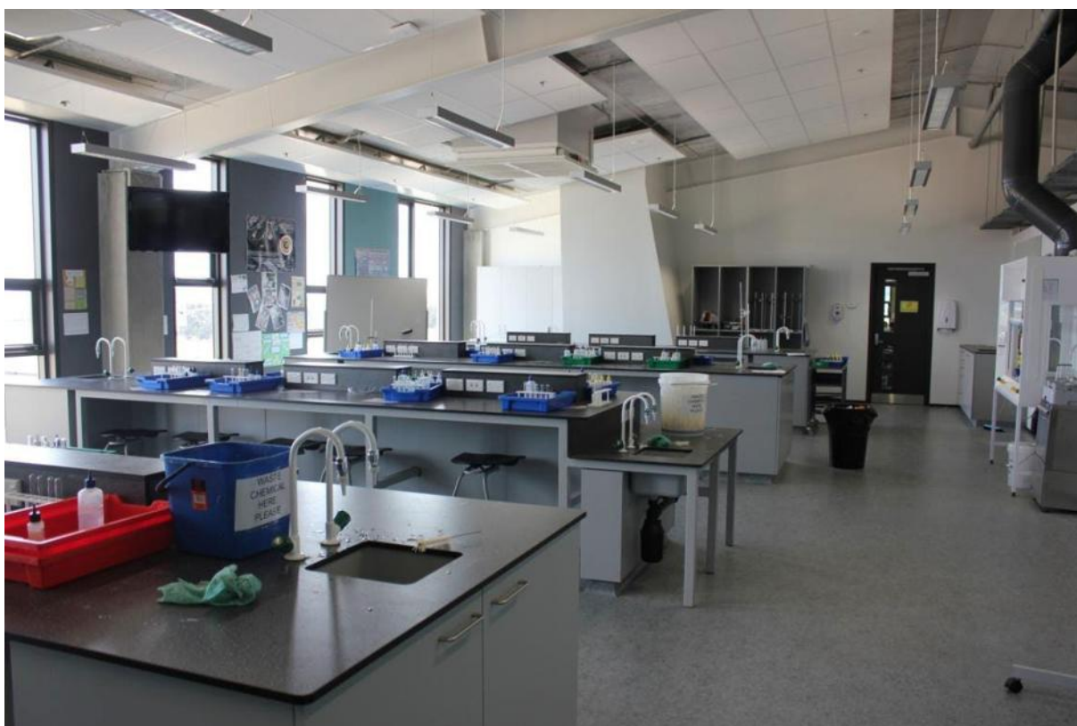
Figure 19: A secondary school science laboratory with fume cupboard and extraction duct
