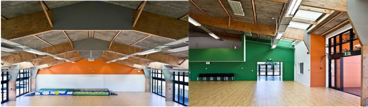
Figure 13: Primary school hall with a simple intuitive design incorporating good cross ventilation through a combination of open doors for warm weather and openable high-level windows for less clement weather. Low-cost electric radiant heating provides quick warming of the space, suited for intermittent use and warm climates.
